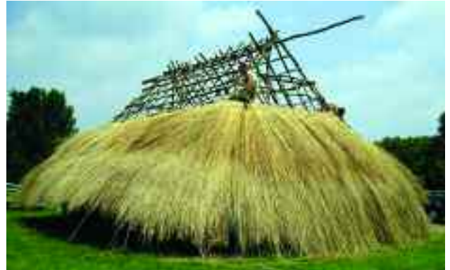
Figure 2: Staff member Shawn McCarty uses native prairie grass to thatch the roof of the ceremonial Big House.
